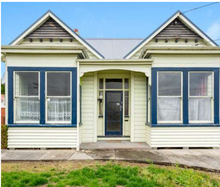
59 Johnson Street, Milton
